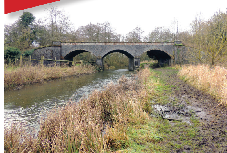
Bridge 1714 over the River Wensum – Part of the rail route at Fakenham now owned by the Melton Constable Trust. Photo courtesy of Tim Horn.
